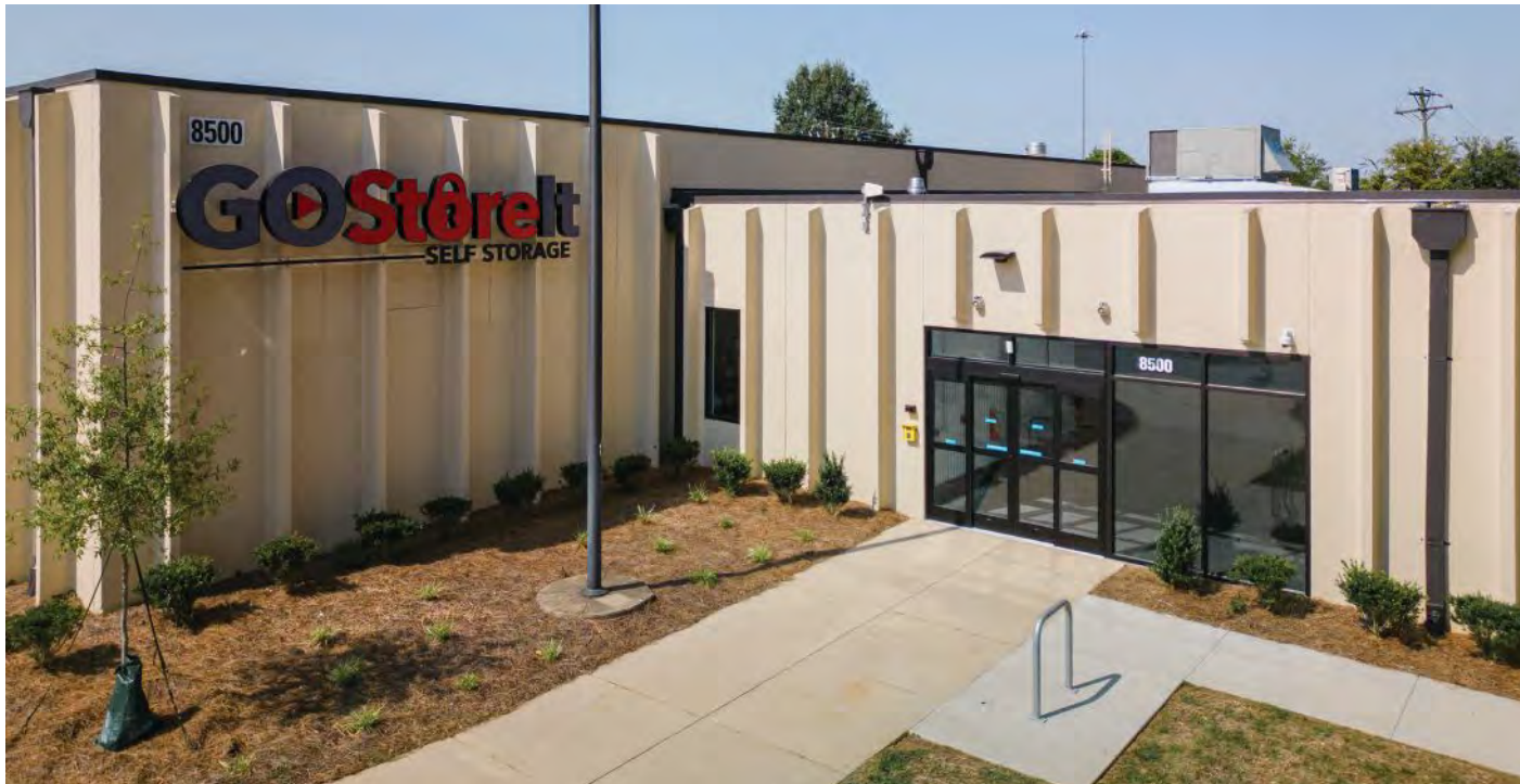
This Go Store It facility in Charlotte was formerly an industrial building. The property was repositioned into self-storage in 2023.
